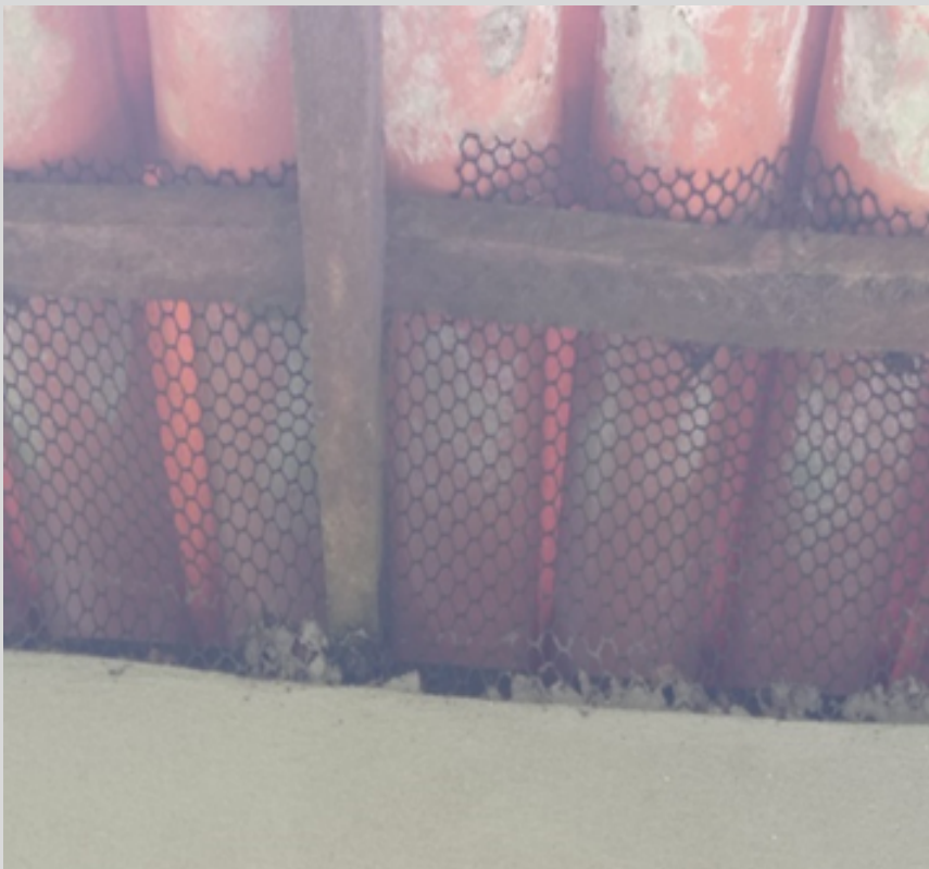
Telar as frestas do telhado
