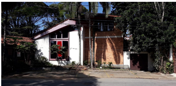
Figure 7: Façade of the old Tobias Clinic on Rua Regina Badra.
