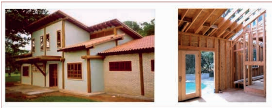
Figure 2 – Examples of contemporary buildings made of wood (left) IBAMA/DF building with pillar-beam system and framed fences in masonry (MELLO, 2004); (right) Typical structure of a house (DON VANDERVORT, 2021).
