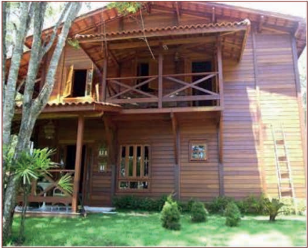
Figure 11 – Finished wooden house, in a pillar-beam construction system
