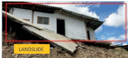
Figure 6. (Top) Wall slightly away from the slide, in red: May scan and in yellow: June scan, (bottom) wall in field.
