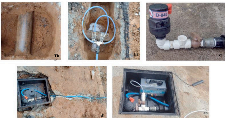
Figure 05 – Box installation on the sidewalk.
