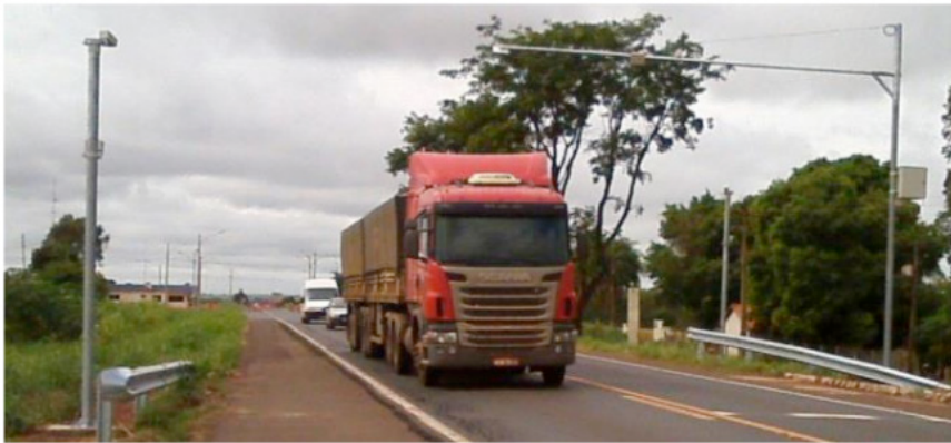
Figura 4: RFID readers installed in the Canal Verde Brasil Project (Barbosa, 2018).
