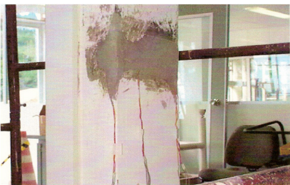
FIGURE 6: Instrumentation of central column reinforcements (recovery after instrumentation)
