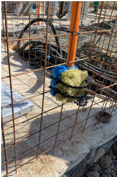
Figure 2 - Rock wool application in electrical boxes before concreting
